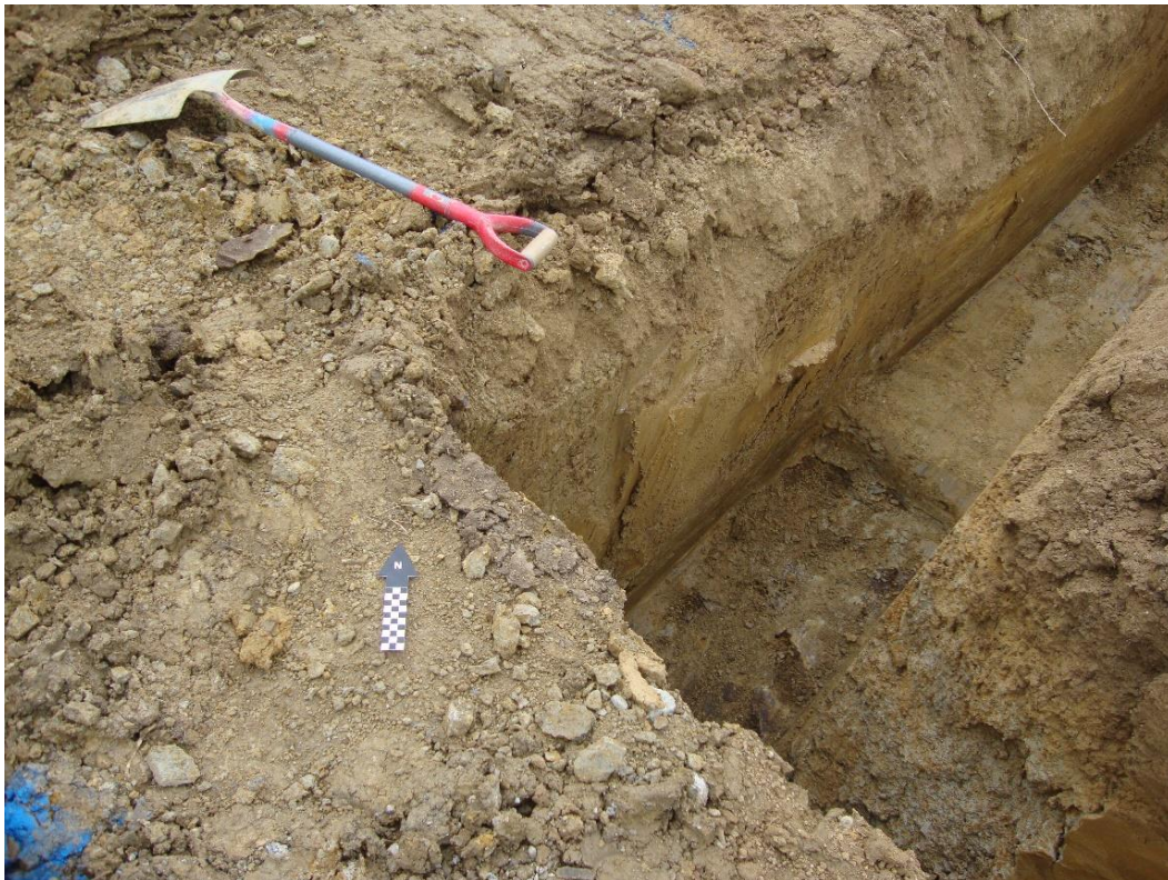
Plate 10. View of foundation trench Plot 8 (looking N)
