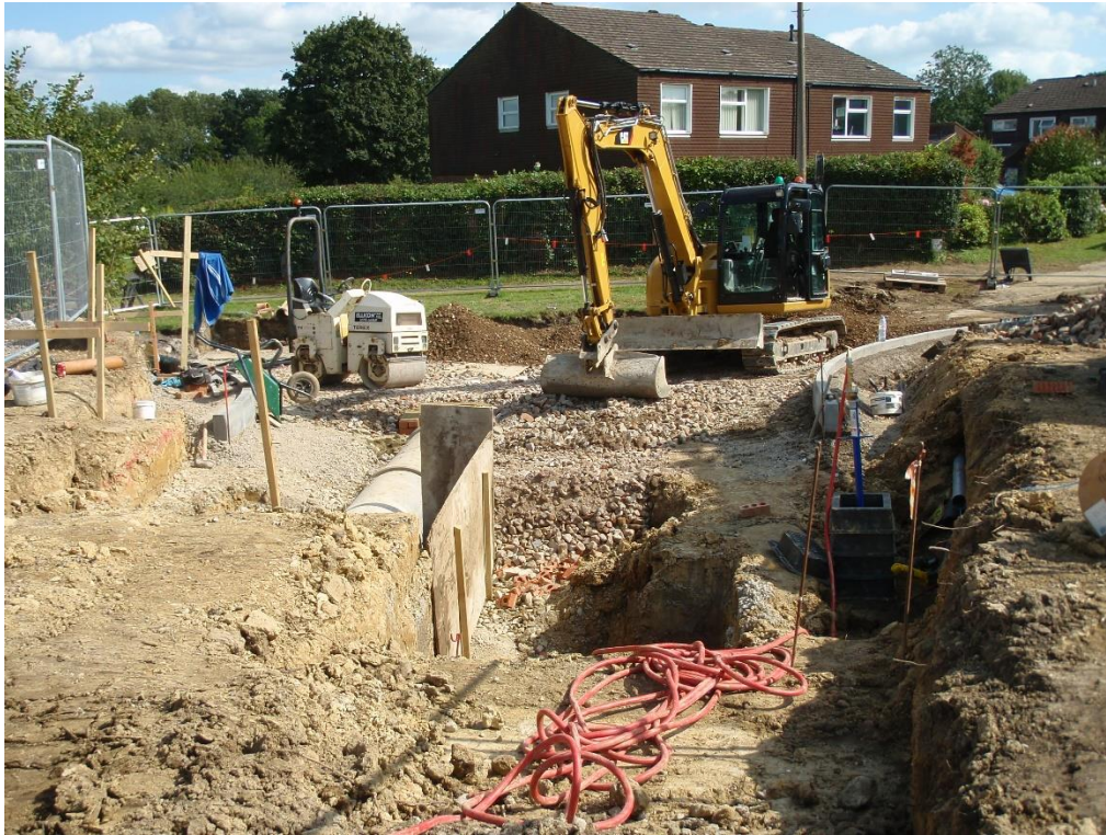
Plate 1. View of the access road and drainage (looking SW)
