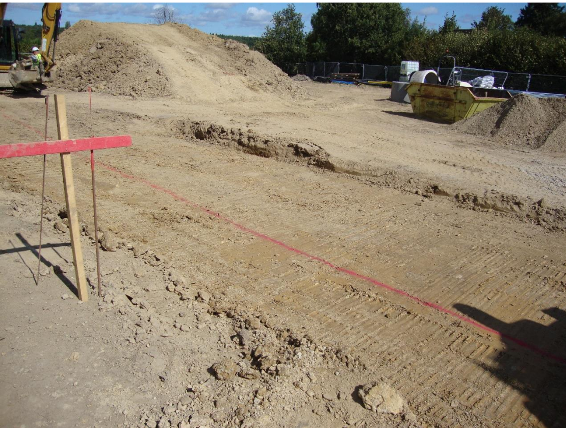
Plate 12. View of access road (looking N)
