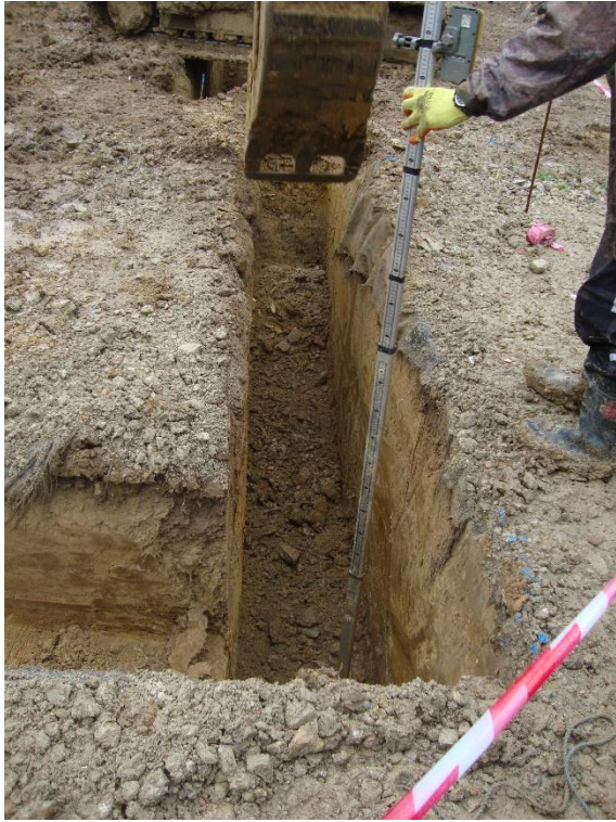
Plate 7. View of Trenches- Plot 7 (looking N)
