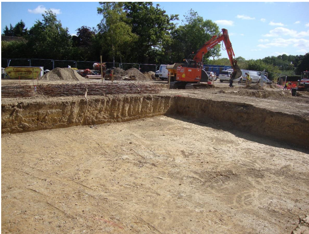
Plate 14. View of excavated areas Plot 6 (looking E)
