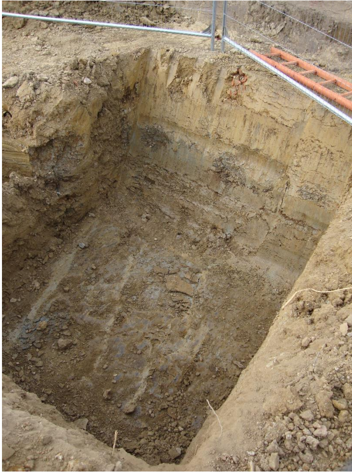
Plate 3. Manhole Pit NW corner- Plot 7
