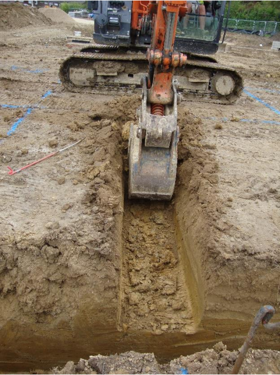
Plate 11. View of foundation trench-Plot 9
